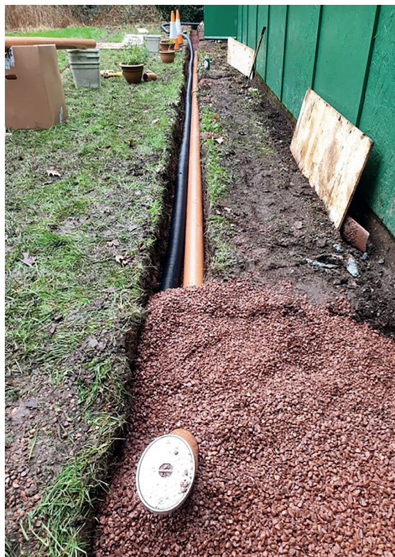
Newly installed drainage to replace old, cracked pipes -fitted thanks to funding from the Community Infrastructure Levy.
