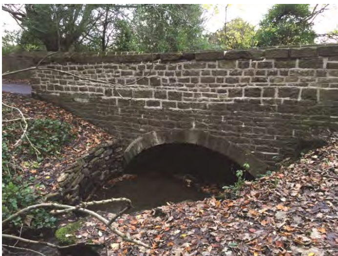
The stretch of Hillfoot Road from the Crown pub up to Old Hay Lane was recently closed to allow the repair, refurbishing and repointing of the two bridges over the streams. The photo above shows the completed work on the bridge over Needham's Dyke near the Crown pub.
