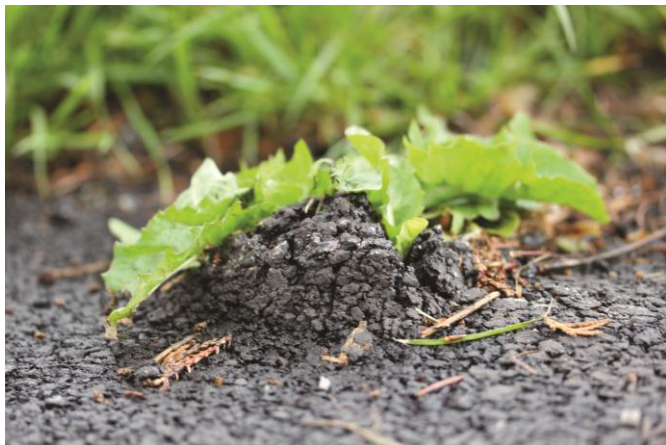
Baslow Road: Weeds erupt from the new pavement tarmac – they will destroy the new surface
